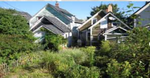
existing buildings from laneway
