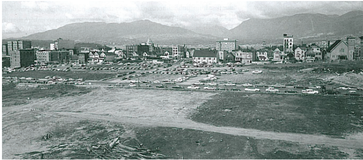
Four blocks of homes demolished in 1968 for construction of a housing project. Source: VPL Special Collections 3235
