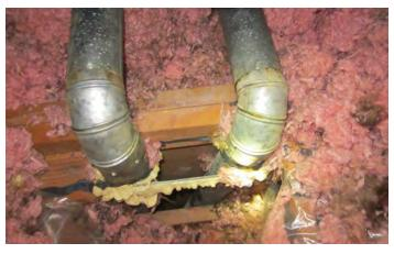
A relatively large hole in the ceiling plane through which two ducts are installed.
