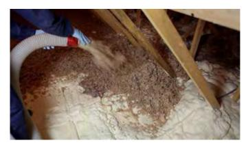
Flash-and-fill attic installation where a few inches of sprayfoam is sprayed to top of ceiling drywall, and then covered with lower cost low-density cellulose or fibreglass insulation fill.
