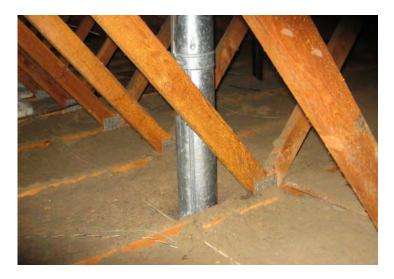
Uninsulated and un-sealed exhaust duct running through an attic, leaking air and heat to the space.
