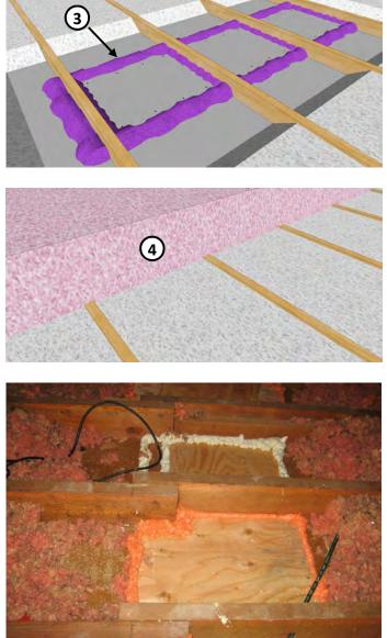
Sprayfoam around the edges of a cover, sealing it to surrounding joists and ceiling gypsum board.
