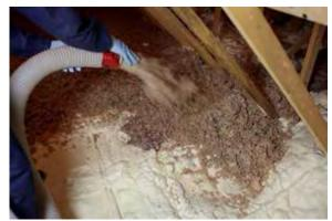
Insulation retrofit of an attic, showing blown-in cellulose added after air sealing and insulating with polyurethane foam.
