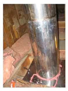
Metal chimney with sheet metal seal over ceiling joists.
