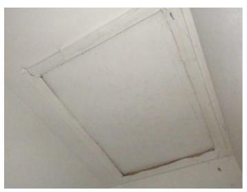
An attic access hatch made from plywood resting on a woodtrimmed opening.
