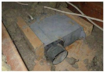
Bathroom exhaust fan venting into the attic. Conditions such as this should be remedied prior to or as part of air sealing and insulation work.
