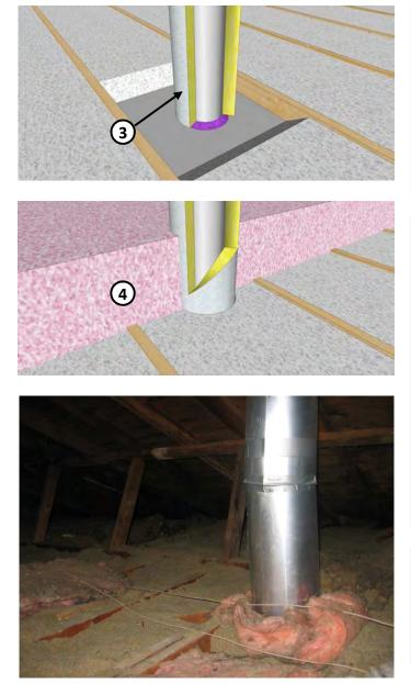
Insulated and sealed exhaust duct in an attic.
