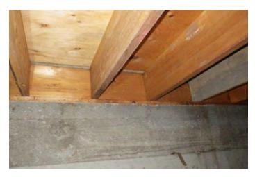
Exposed below-grade wall at floor rim joist.
