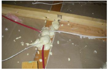
Top plate penetrations sealed with sprayfoam.
