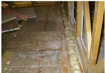
Sprayfoam installed over top plate joint.
