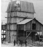
**Photo:** c1888, Vancouver, San Juan Lime Co. kiln - many such works were erected in the colonial period to burn limestone and make quicklime (CaO) from which lime mortar was produced. BCA HP009184
