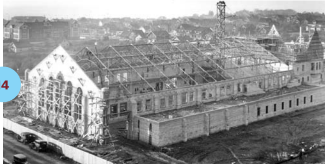
Seaforth Armoury under construction 1935 (Matthews) Bu P794.2
