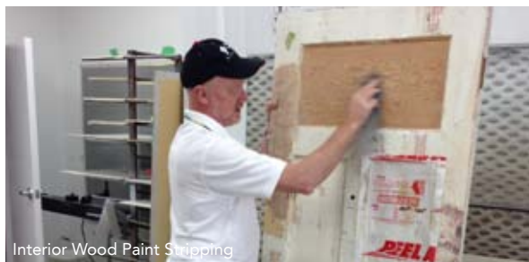
Interior Wood Paint Stripping
