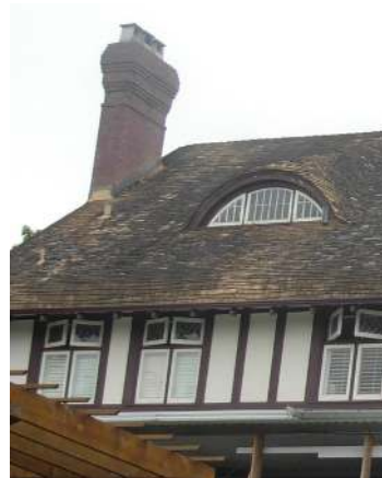
5055 Connaught Dr Brooks House 3rd Shaughnessey Replacement rolled shingle roof, 2008 Heritage Register: A(M)(H)(L)
