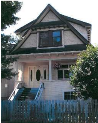
1784 E 14th Ave John Tibb House Trout Lake New gutters, beveled glass entry door restoration, 2012 Heritage Register: C(M) Built: 1912
