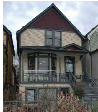
827 E Georgia St Hendrix House Strathcona Restoration of front porch and stairs, 2007 Heritage Register: C(M) Built: 1904
