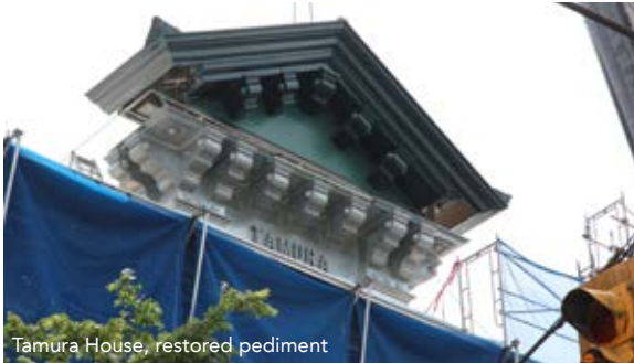
Tamura House, restored pediment
