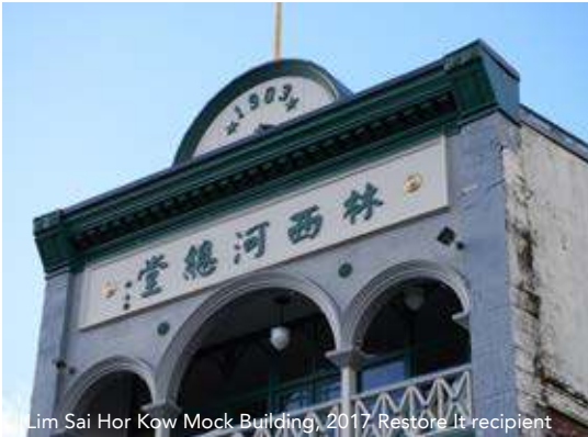
Lim Sai Hor Kow Mock Building, 2017 Restore It recipient
