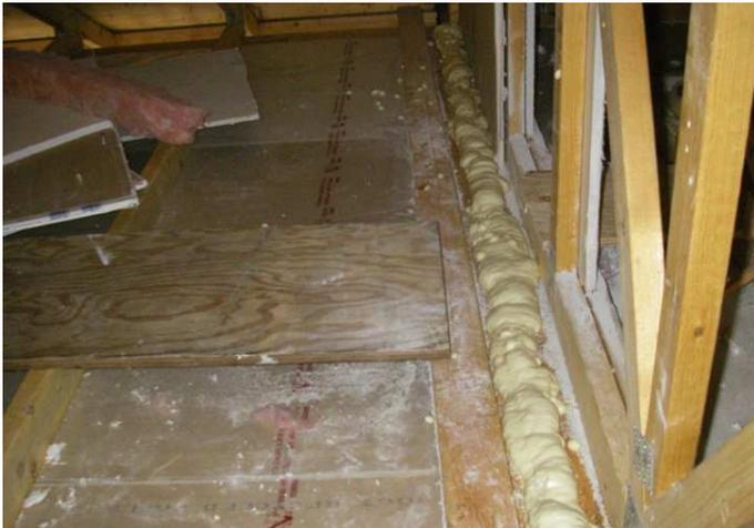
*Sprayfoam installed over top plate joint.*
