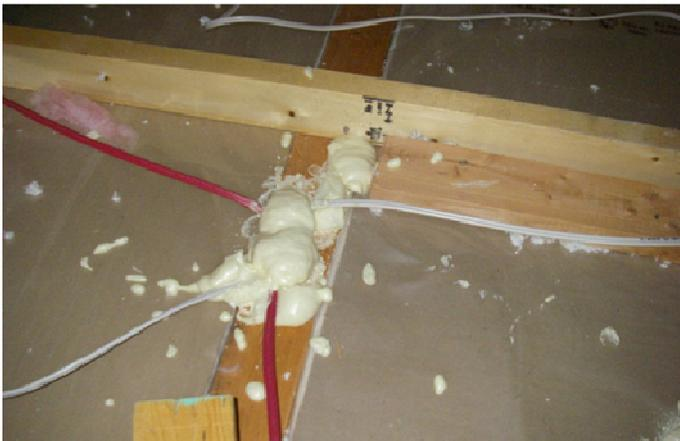
*Top plate penetrations sealed with sprayfoam.*
