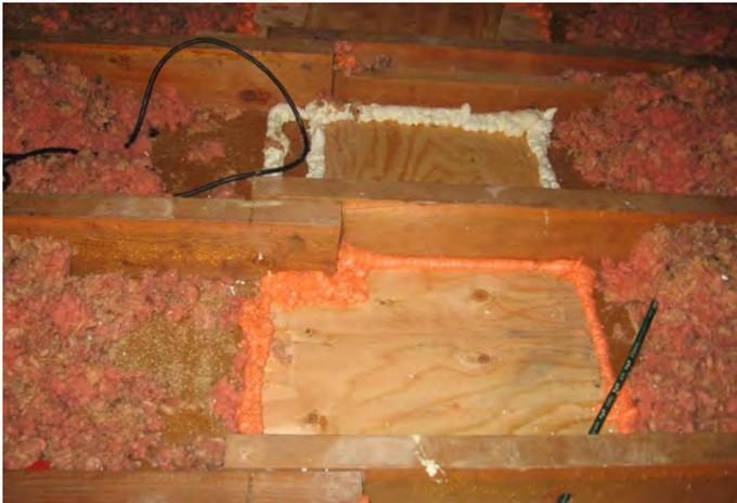
Sprayfoam around the edges of a cover, sealing it to surrounding joists and ceiling gypsum board.
