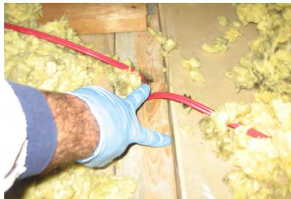
*Air sealing of an electrical penetration and unsealed top-plate connection in an attic.*
