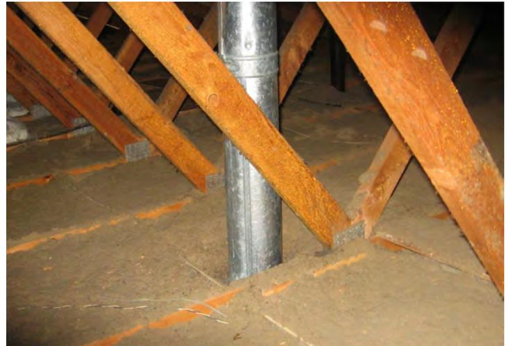
*Uninsulated and un-sealed exhaust duct running through an attic, leaking air and heat to the space.*
