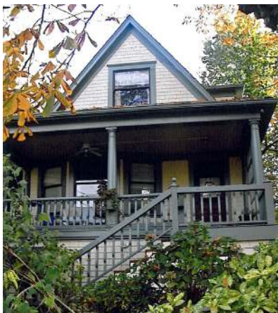
1928 Stephens St Painted: 2011 Style: Edwardian Built: 1908 Heritage Register: C
