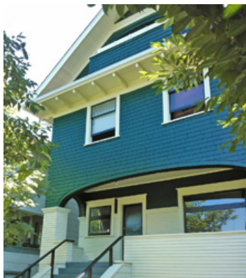
3550 W 1st Ave Painted: 2013 Style: Craftsman Built: 1917 Heritage Register: C
