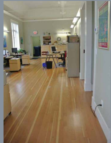
■ Finished and reconfigured interiors of the Barn, with drop ceiling removed and original wooden flooring in place
