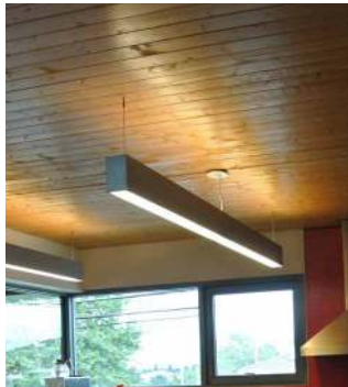
Flooring is repurposed as ceiling paneling in the kitchen and stairwells
