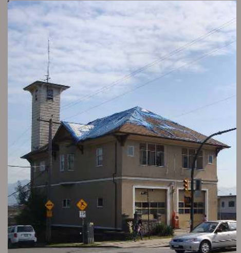
■ The fire hall prior to its restoration, with blue tarps covering the roof where its surface was failing.
