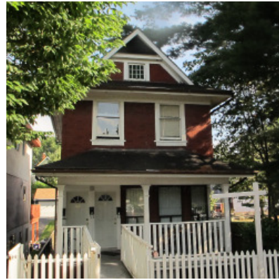
777 Union Street Strathcona The Lawler House Built: 1908 Style: Edwardian Heritage Register: C
