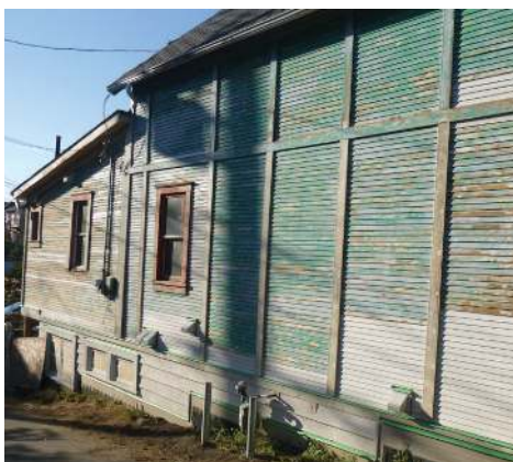
Building Face Repair: Much of the siding on this historic house was in need of either repair or replacement prior to painting, but overall remained intact.
