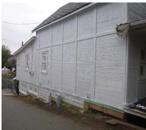
Building Face Repair: Much of the siding on this historic house was in need of either repair or replacement prior to painting, but overall remained intact.
