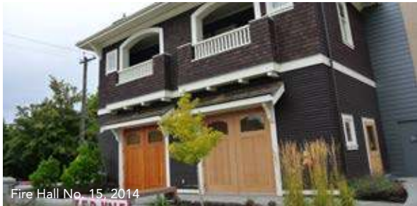
Fire Hall No. 15, 2014
