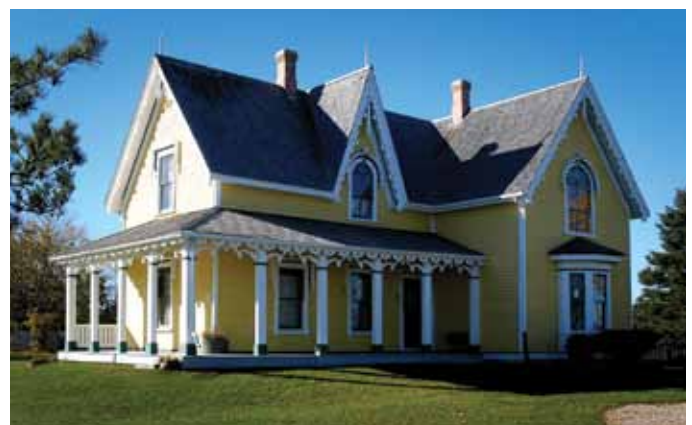
Based on documentary evidence, including an 1880 engraving, the original fenestration of the Bideford Parsonage Museum in P.E.I. was restored and roof finials replaced.
