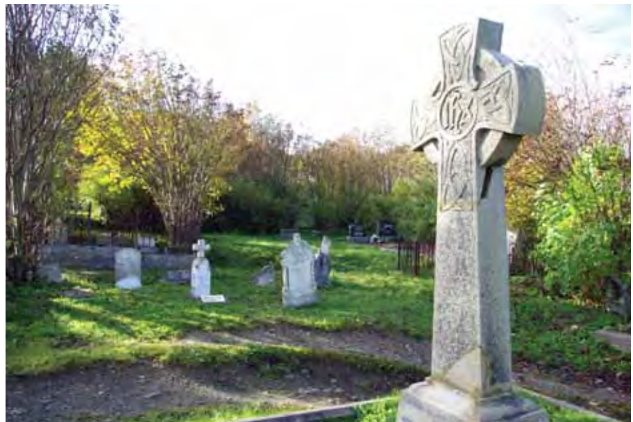
A condition assessment and evaluation undertaken before an intervention at Belvedere Cemetery in St. John's Ecclesiastical District, would reveal that the well-aged and weathered patina found on the grave markers is not damaging. It is in fact a character-defining element of this historic place and should be preserved.
