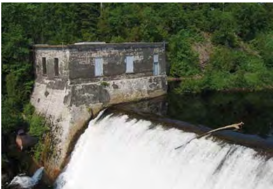
Remains of hydroelectric installations.
