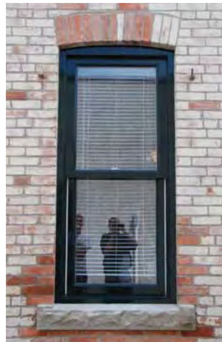
Left: North façade window prior to rehabilitation showing eroded mortar joints, cracking due to frost action within the wet wall, and delamination of the sandstone sill.
