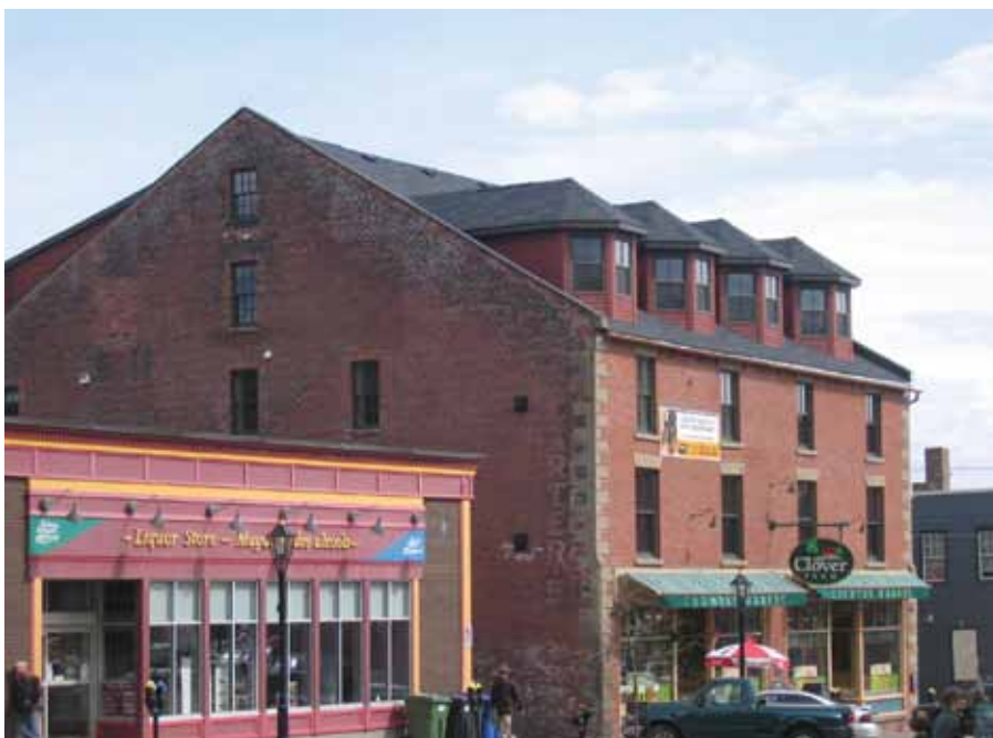
In order to accommodate new condominium units in the upper floor of this building on Queen Street in Charlottetown, new dormers were added. In Rehabilitation, the design of new elements should be compatible with the heritage value of the historic place.
