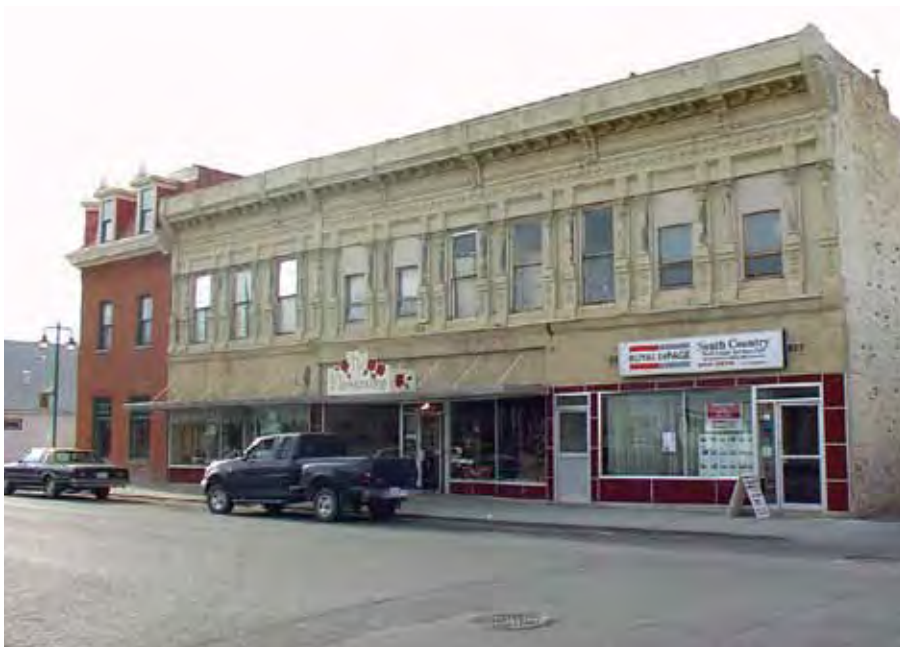
Before rehabilitation: east façade, looking southwest.
