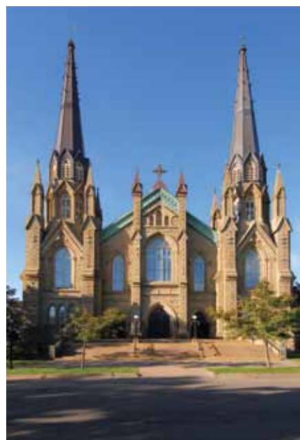
It is important to consider the expected life span of all elements that make up a roof assembly when repairing or replacing a roof such as this one on St. Dunstan's Basilica in Prince Edward Island. Roofing materials, such as copper and slate, need to be matched with flashings of a similar life span.
