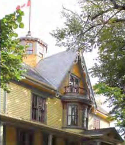
When the windows of Lefurgey House in Summerside, PEI were damaged in a fire, instead of replacing the entire windows, only the broken glass was replaced. The replacement glass, salvaged from a nearby house that was replacing its windows, had similar properties and wavy appearance.
