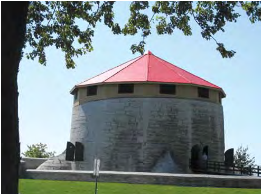
Murney Tower, in Kingston, ON, is a martello tower that forms part of the defence system built for Kingston Harbour during the Oregon Crisis of 1845–1846. It is a squat round tower with four hive-like caponiers at its base and a conical roof and is surrounded by a dry ditch. Murney Tower is valued for its excellent portrayal of the martello tower military structure, its built and landscaped forms, and also its strategic setting and defensive inter-relationship with other parts of the Kingston Fortifications.
