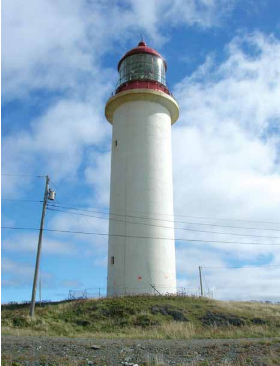
Cape Race Lighthouse, on the southernmost tip of the Avalon Peninsula in Newfoundland and Labrador, is Canada's most prominent landfall marker. Built in 1906–1907, Cape Race was the first Canadian lighthouse to be constructed in reinforced concrete and probably the second lighthouse constructed in reinforced concrete in the world.
