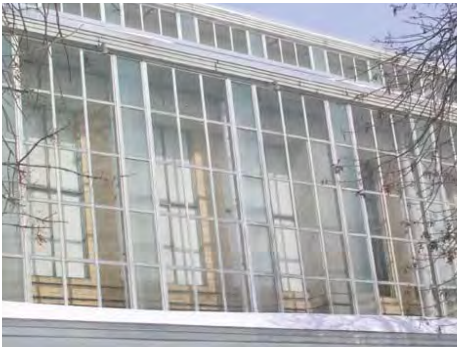
The character-defining transparency of the glass-enclosed factory wings of the National Printing Bureau in Gatineau, QC was preserved during conservation work on the glass and aluminium curtain walls. After the thin aluminium frames were cleaned, the opaque ribbed glass and clear plate glass were carefully reset in their original positions that reflect the pattern of solids and voids in the masonry wall behind.
