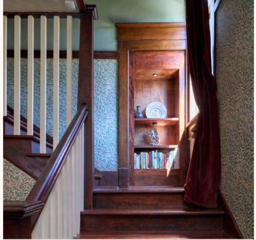
View of historic domestic stairs (leading to the kitchen) adapted by the current owners into a bookshelf
